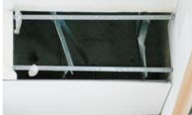
Walls of the ceiling and side came off.
