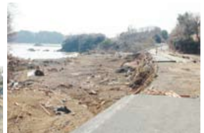
National Highway 45 just after the earthquake.
