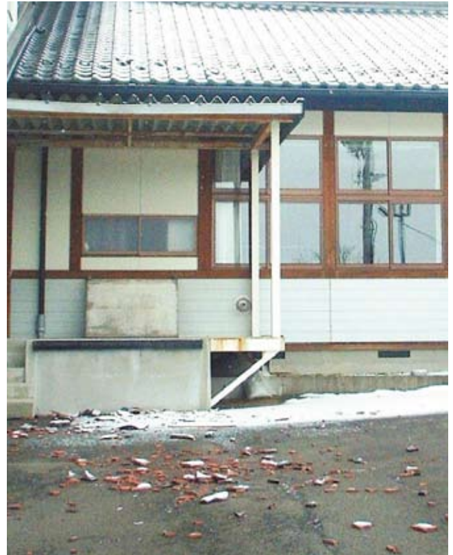
Roof tiles dropped
