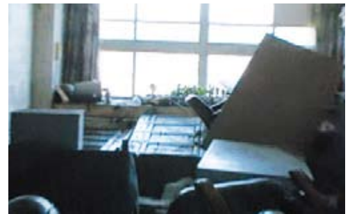
The situation of the inside of a principal's room looked at from a passage. A bookshelf and a safe fell down sideways in the tsunami.
