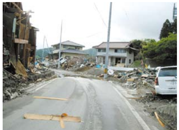
Main road faced to be submerged and collapsed
