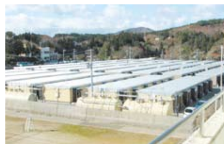
Temporary dwellings in the playground. 186 apartments.
