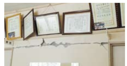
Cracks of the corridor
