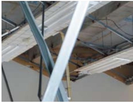
Ceiling board of the music room fall down
