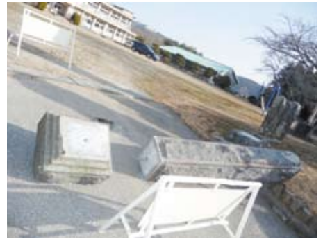
Destruction of the cornerstone of school gate
