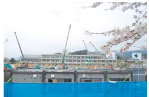
Temporary housing being constructed in the schoolyard.
