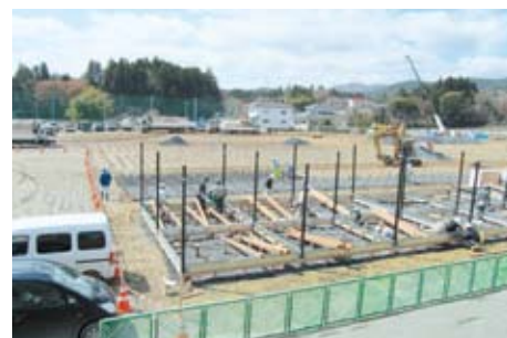
Beginning of construction of temporary houses in the schoolyard.
