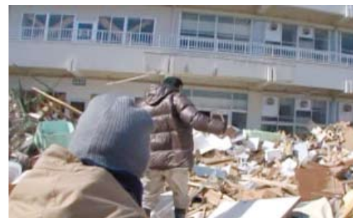
This is the situation of the front of a staff room (the school ground). Rubble (cars and demolished houses) are piled high.
