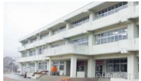
The school building of Ohya Junior High School in April.
