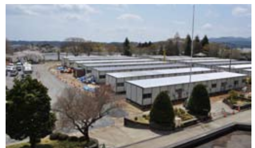
The other side, temporary housing (on April 28)
