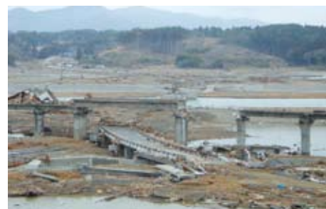
A washed out bridge and collapsed railroad line.
