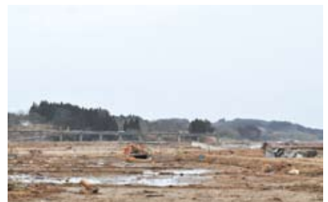
1.5 km from the river's mouth: the railway of the Kesenuma line which had been on the bridge and was driven away.
