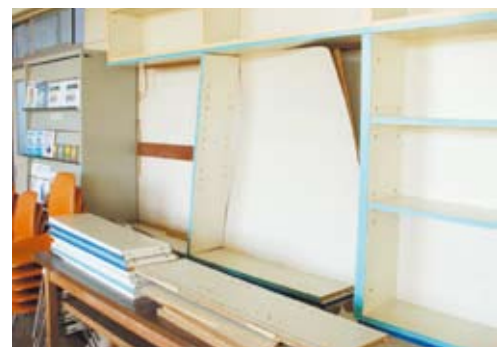
Library damage due to the earthquake.
