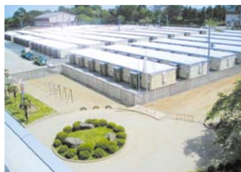
186 Temporary Houses at School Ground
