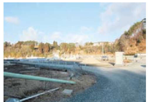
Around Kosaba Port, suffering from the most serious damage in the school district: the villages along the coast were completely destroyed by tsunami. A temporary embankment was built with the sandbags on the coastline, and the roads were raised.
