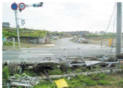
Destruction State of Ohya Kaigan Station
