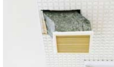
The room could not be used due to the falling of four air ducts.
