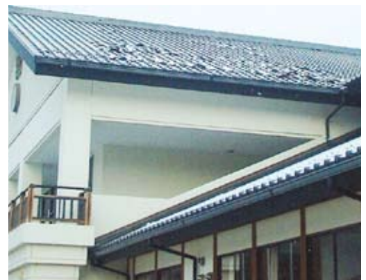
Broken roof tiles
