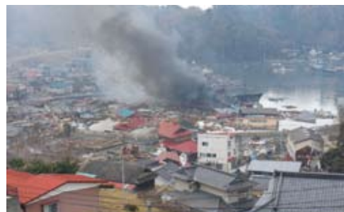
View of the damage in our school district.
