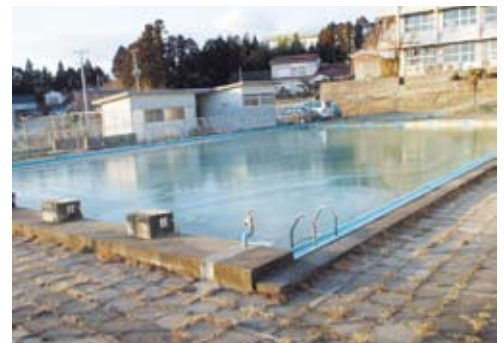
Using the pool water after cleaning up
