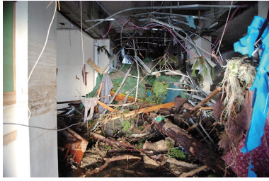
1st floor of the Arahama Elementary School that filled with tsunami debris on the day after the tsunami attack.(Provided by the Center for Remembering 3.11; Sendai Mediatheque).
